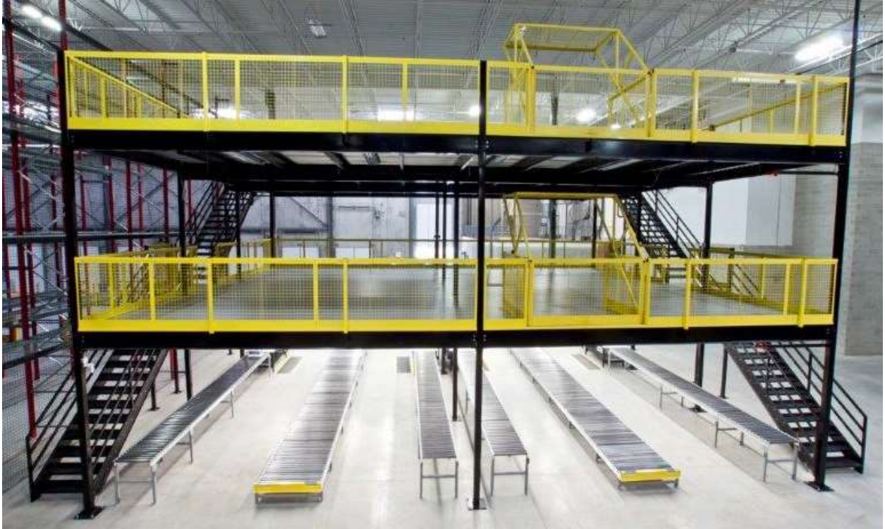
Completed 2-Tier Mezzanine with Stairs and Teeter Gates
