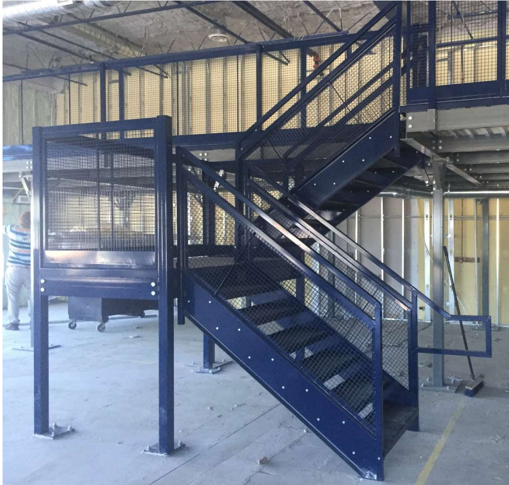
Side View of Installed Stairs
