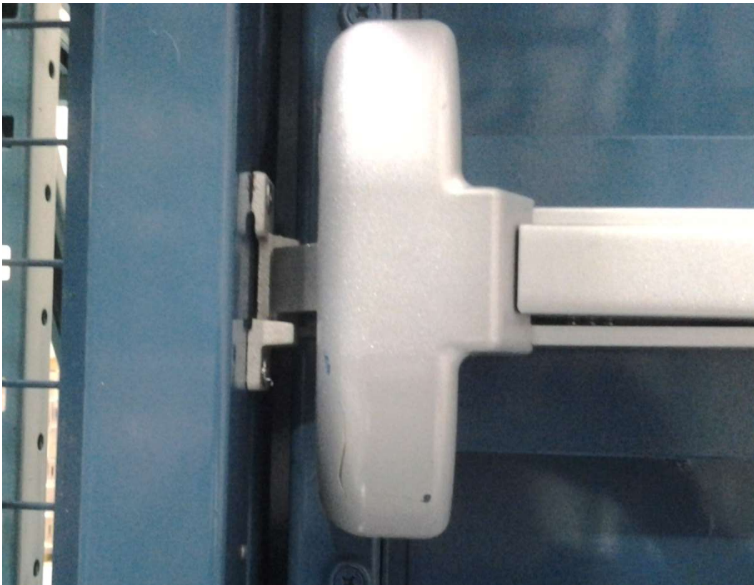
Inside View of Panic Bar Strike Installed
