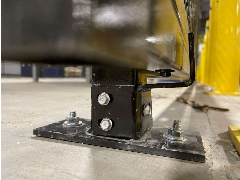
"Z" Guide Installed
